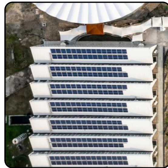
SECURE METERS LIMITED (Sanand GIDC, Gujarat, India) 420 kWp
